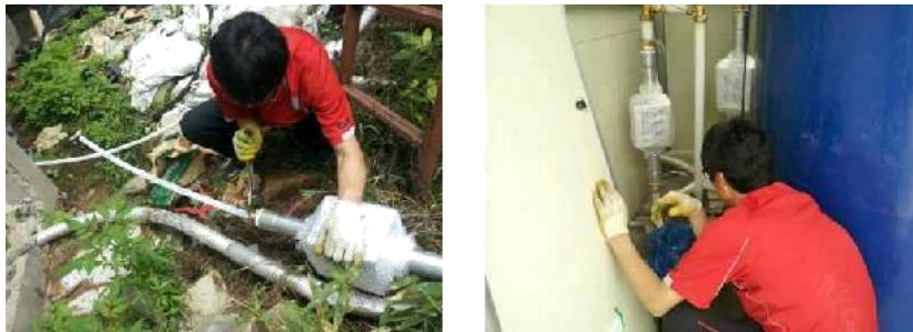
Fig 1. Installation of magnetic instrument
